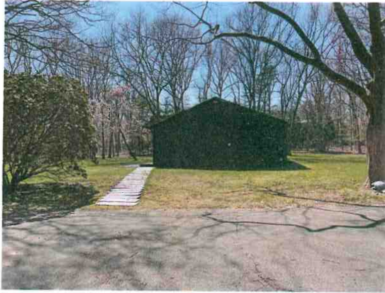
Existing One-Story Residence
